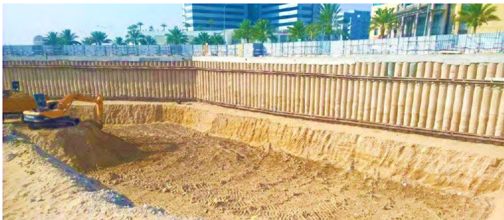
Figure 5-202 Piled wall example
