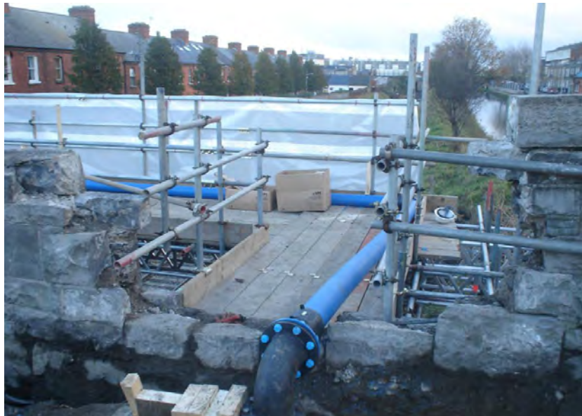
Figure 5-7 Temporary diversion along scaffolding
