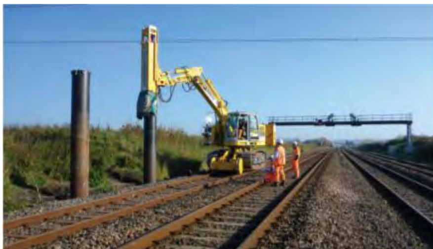
Figure 5-79 Installation of steel piles
