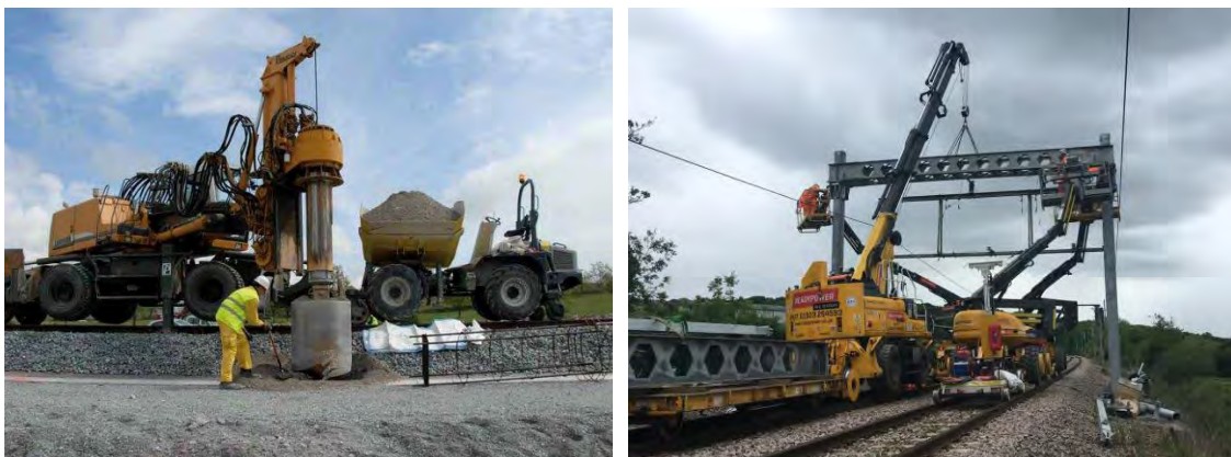
Figure 5-73 Rail-road vehicle examples - pile boring machinery (left) and crane (right)
