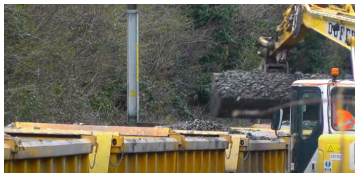
Figure 5-15 Ballast removal
