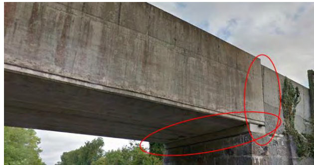
Figure 5-390 Joints to be demolished at abutment
