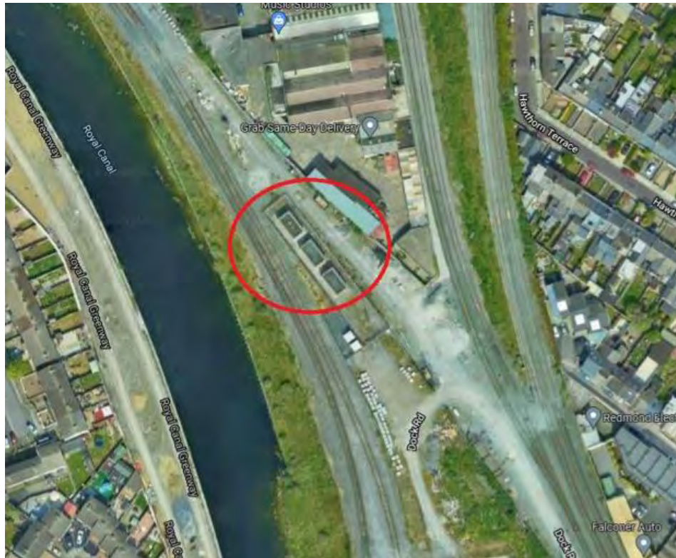
Figure 5-222 Existing technical buildings
