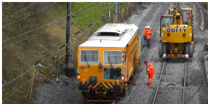
Figure 5-22 Ballast tamping
