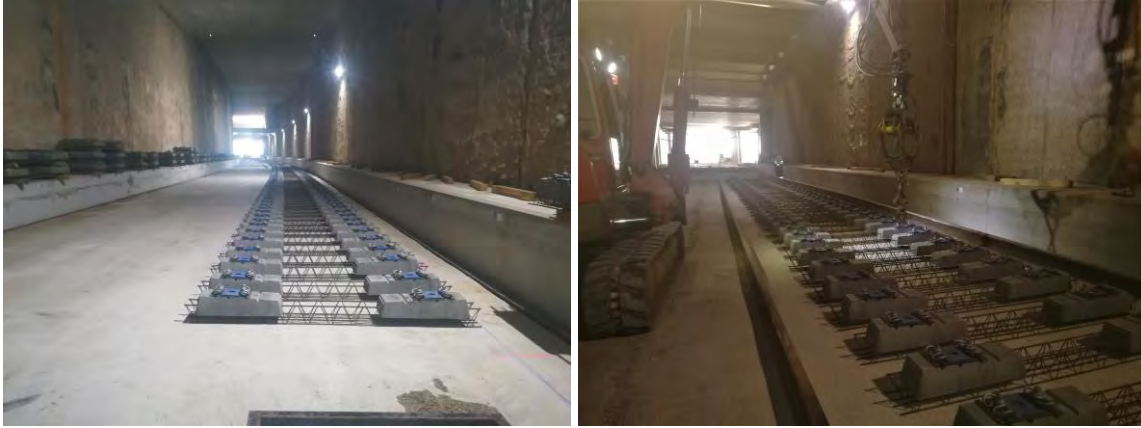
Figure 5-29 Sleeper laying on top of structural slab
