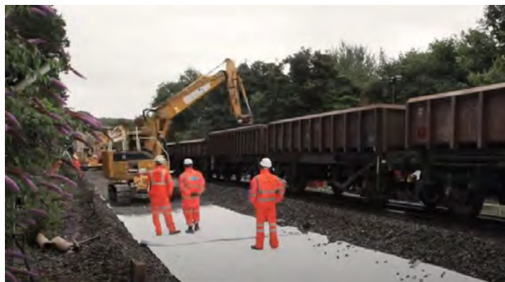
Figure 5-17 Ballast laying
