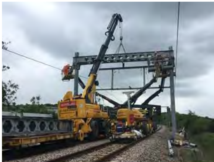
Figure 5-82 Gantry installation
