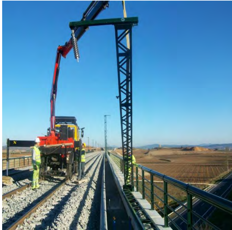
Figure 5-81 Mast installation
