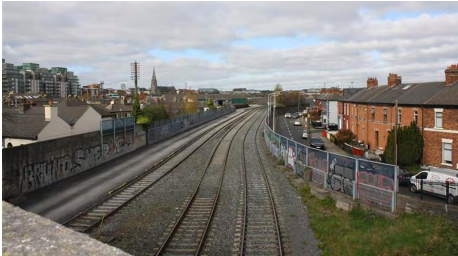
Figure 5-132 Dock Road showing live rail interface
