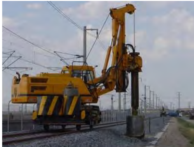
Figure 5-77 Foundation drilling
