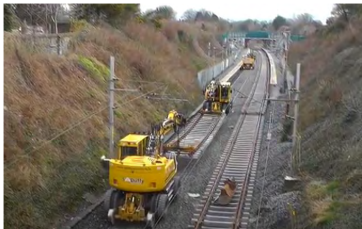
Figure 5-14 Track panel removal
