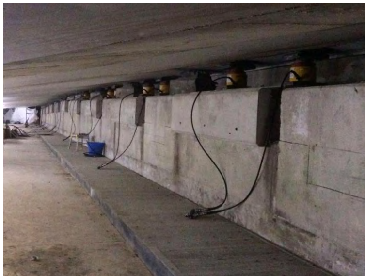
Figure 5-56 Standard bridge jacking system
