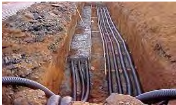
Figure 5-63 Example of buried ducts for substation connections
