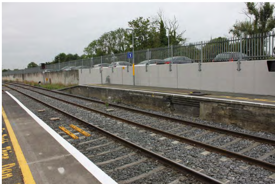
Figure 5-338 End of east platform (Platform 1)
