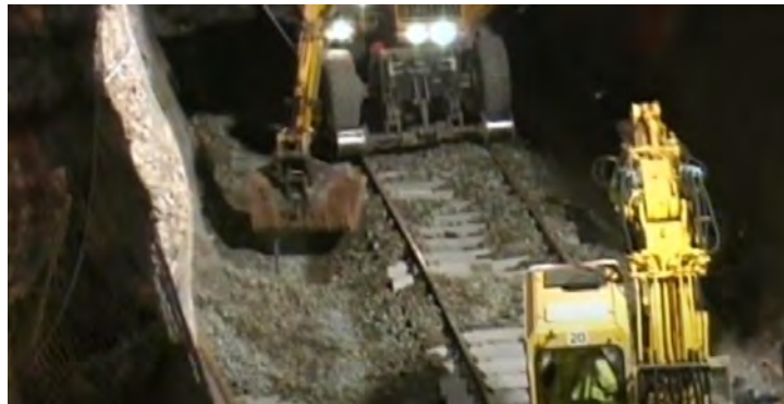
Figure 5-21 Ballast laying – second layer
