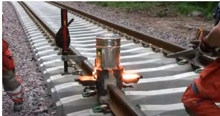
Figure 5-23 Rail joint welding
