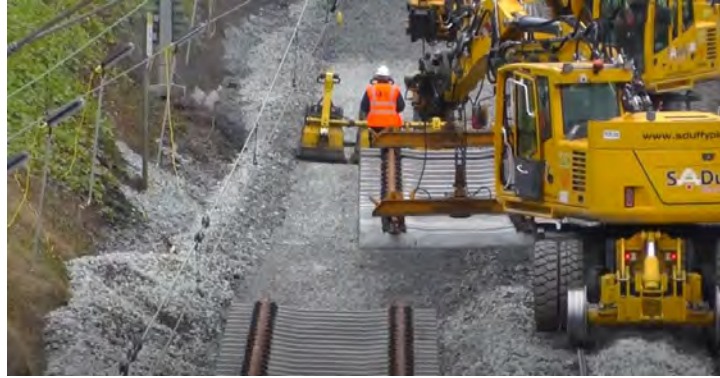
Figure 5-19 Track panel installation
