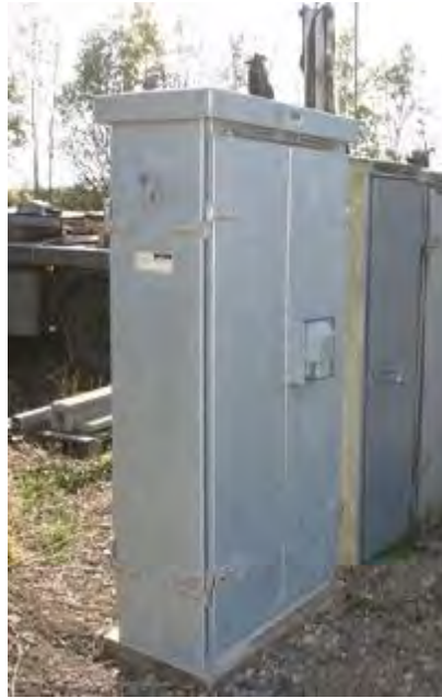
Figure 5-72 Typical LOC (location case)
