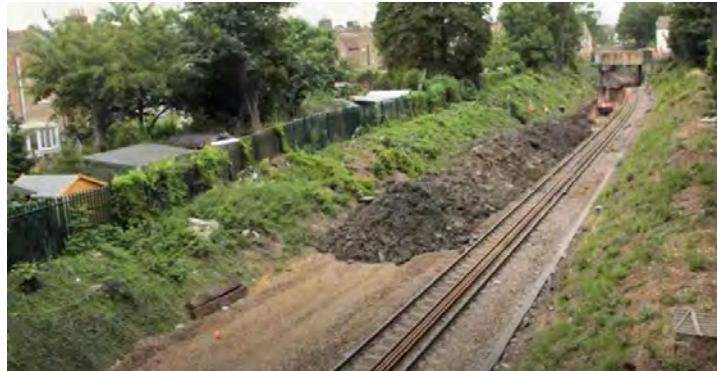
Figure 5-16 Platform excavation
