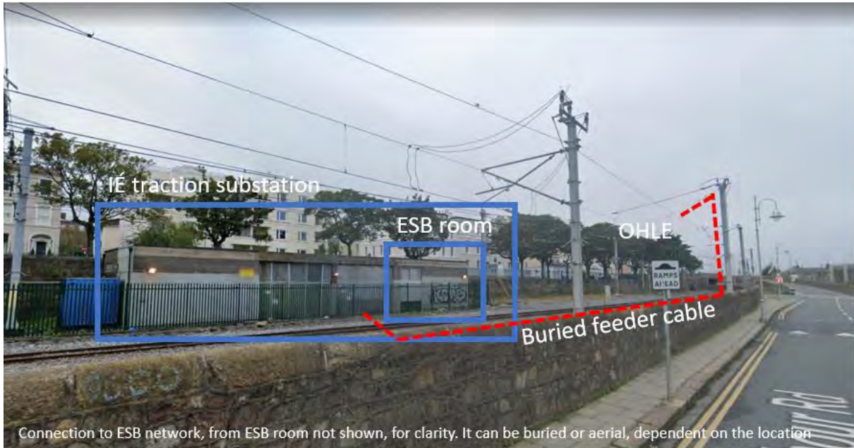
Figure 5-62 Traction substation connections
