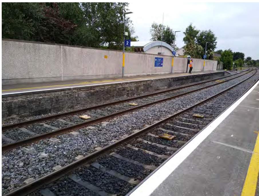
Figure 5-336 End of west platform (Platform 2)
