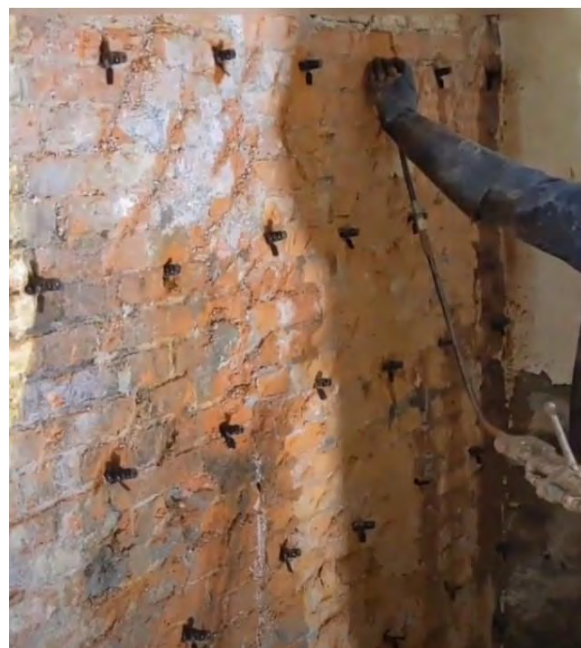
Figure 5-114 Injection of acrylic resin into vaults
