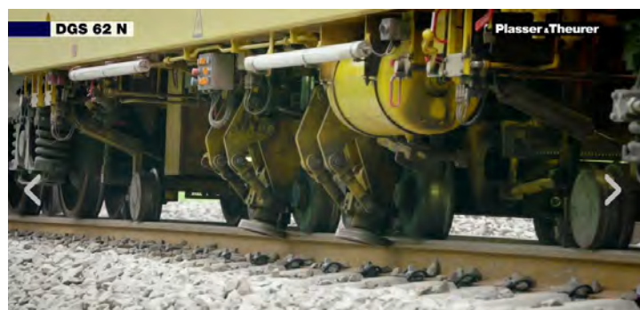
Figure 5-27 Extension of second ballast layer, tamping and dynamic stabilisation
