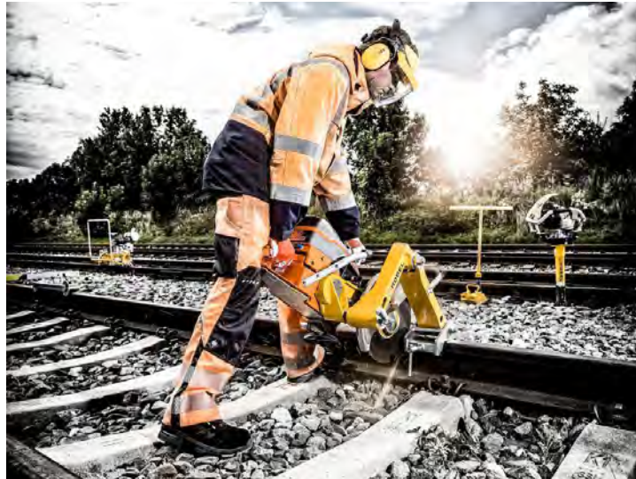
Figure 5-13 Rail cutting
