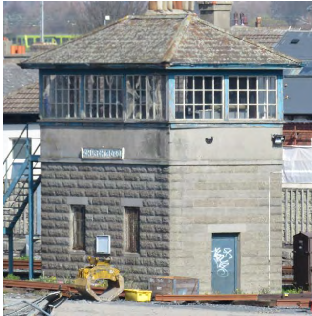
Figure 5-213 Church Road signal box to be demolished
