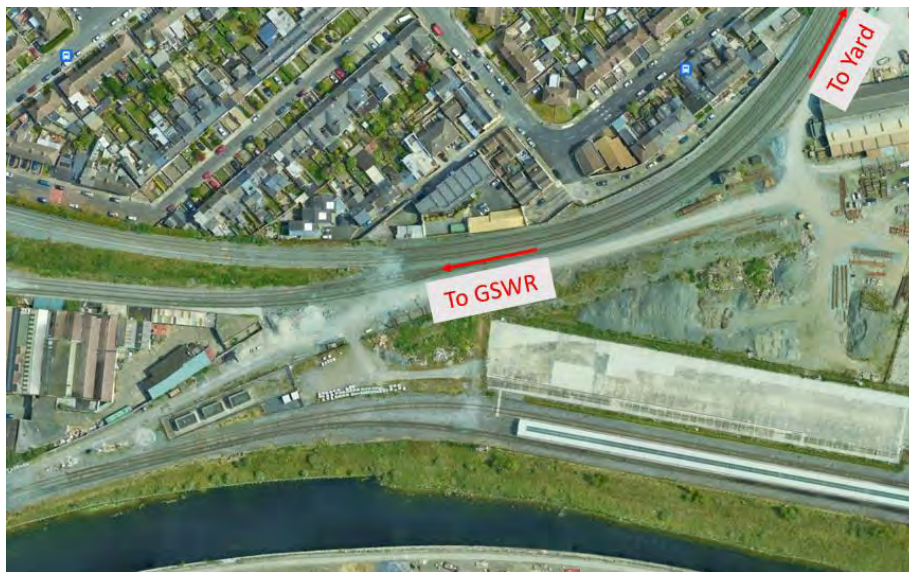
Figure 5-205 Existing GSWR-East Wall yard connection
