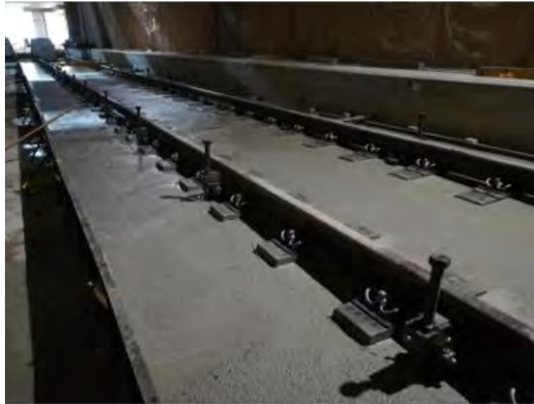
Figure 5-32 Concrete curing
