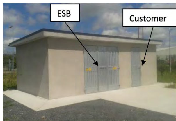
Figure 5-64 Example of MV substation
