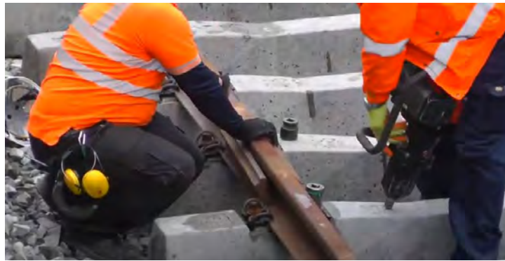
Figure 5-20 Provisional track panel joint
