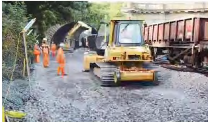
Figure 5-25 Ballast laying and compaction
