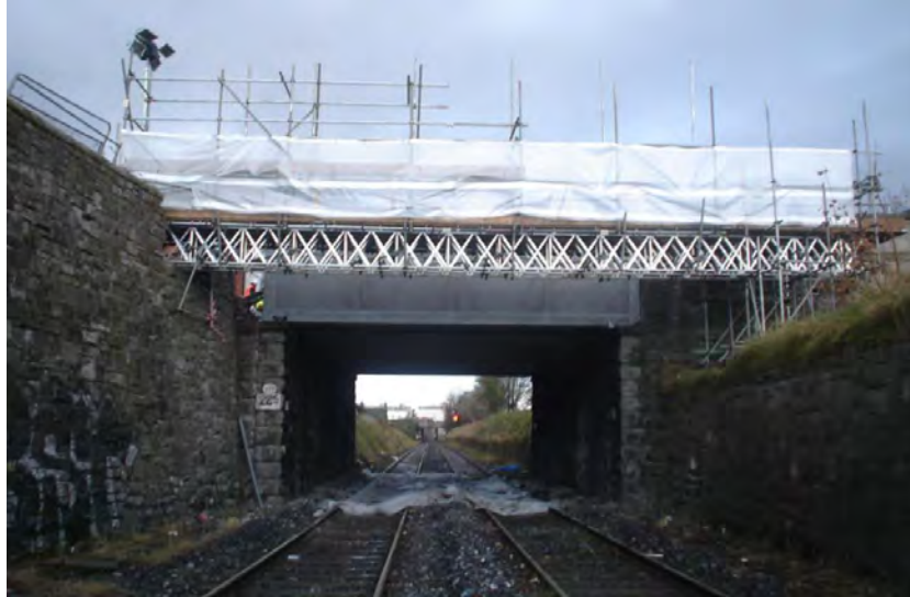
Figure 5-6 Scaffolding for temporary diversion
