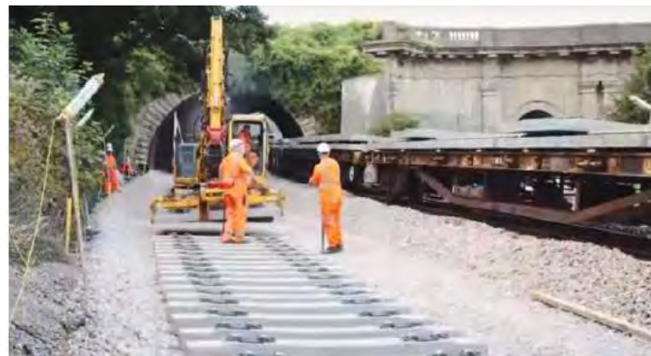
Figure 5-26 Sleeper laying
